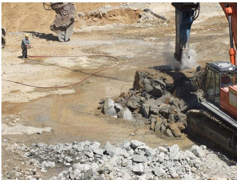
Rubblization in action: pummeling concrete into a base for new roadways.
